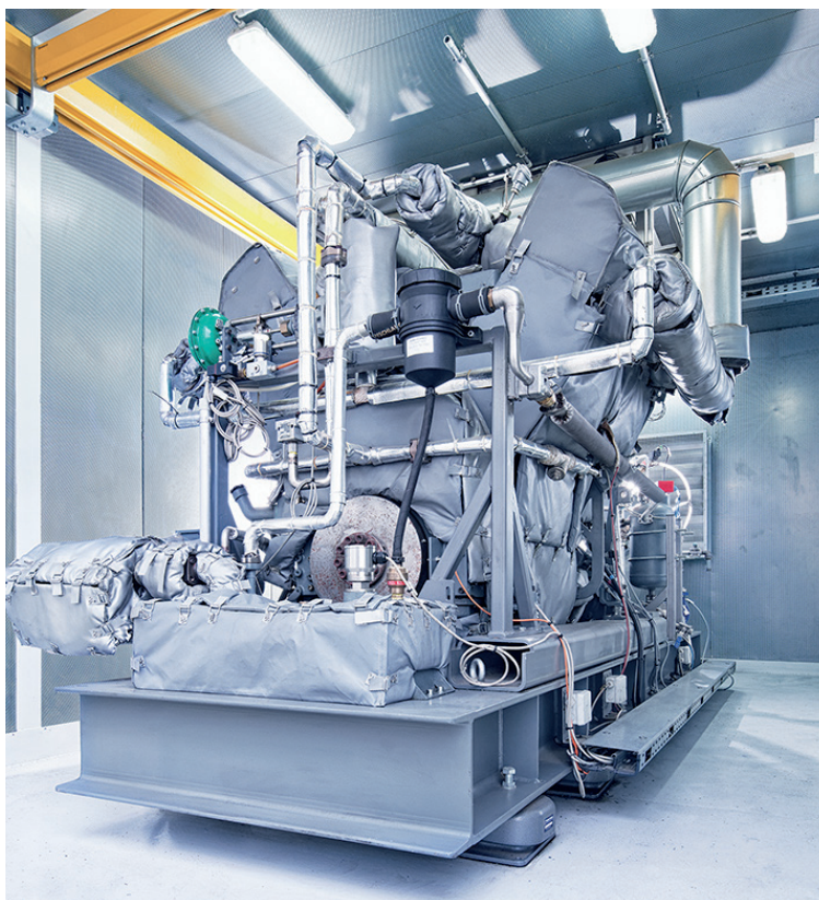
The heart of the ORC unit – a 12-cylinder electricity generation engine
