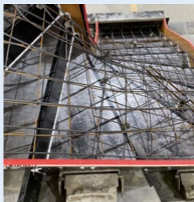
Reduced reinforcement when producing half-turn stairs using STABILS steel fiber (right)
